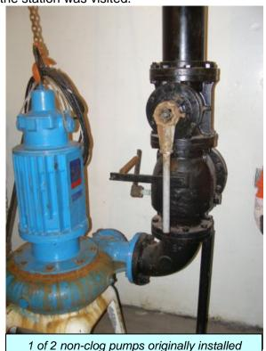
The original non-clog pumps had provided acceptable service when they had been installed about 10 years earlier. But the changing nature of today's sewage, carrying ever increasing amounts of debris such as disposable floor wipes, has rendered these pumps ineffective. The floor wipes and other
