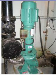
station. The photo below shows the pumps that were installed in the Borst Park pump station in November of 2009. These are 30 HP units rated at 1100 GPM. This year the Military Road, Scammon Creek and High Street lift stations were upgraded to Vaughan
