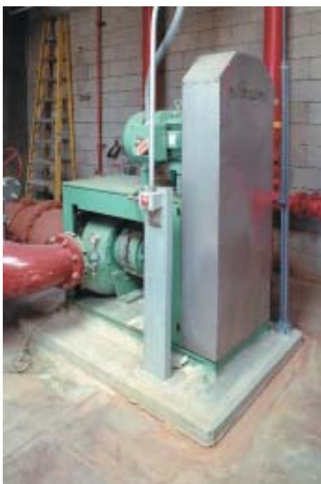
**The Pump** - Vaughan's chopper pump is the *heart* of the Rotamix system, including a patented chopping design, wear parts heat treated to 60+ Rockwell C Hardness, oversized shafting and bearings, heavy duty mechanical seal and back pull-out design.
